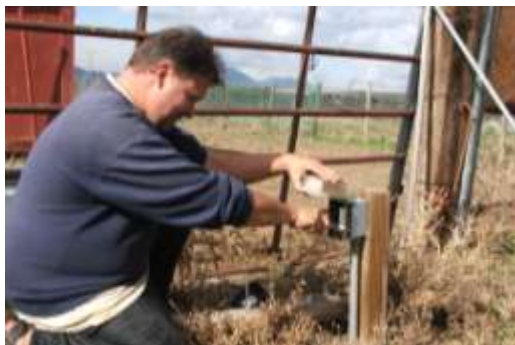
"SPARKY" AKA JEFF MARSHALL , working on the electrical at the rescue
