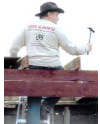
Ray Salinas repairs a roof on a horse shed
