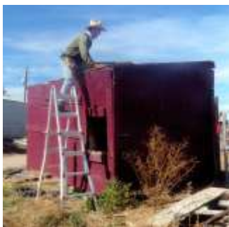
Rob Nixon applies a new roof to a wind-damaged shed
