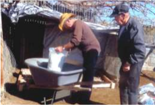
RAY SALINAS AND HANK BALDWIN BUILD A NEW DRY PLATFORM FOR LITTLE BIT'S SHED. THEY BUILD A frame, fill with coarse rock and cover with a rubber mat
