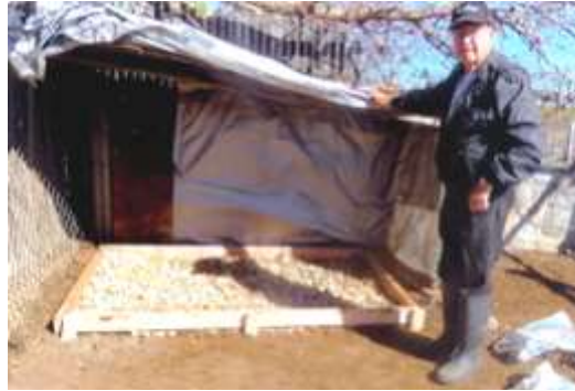
RAY SALINAS AND HANK BALDWIN BUILD A NEW DRY PLATFORM FOR LITTLE BIT'S SHED. THEY BUILD A frame, fill with coarse rock and cover with a rubber mat
