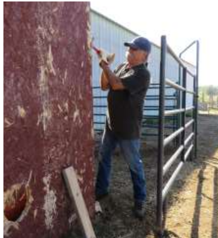
Bily Santiago Repairs a shed
