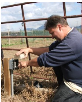
JEFF MARSHALL FIXES AN ELECTRICAL OUTLET THAT IS "ACTING UP"
