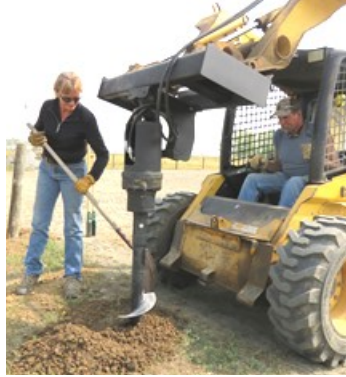
KRIS NIXON SHOVELS WHILE BILL POLZIN DIGS POST HOLES WITH HIS SKID STEER FOR THE CLAIRE DAVIS MEMORIAL ARENA
